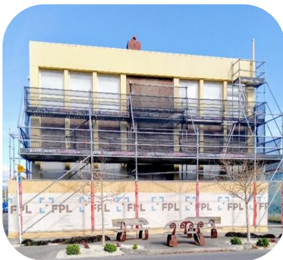
Scaffolding in place in July 2024
